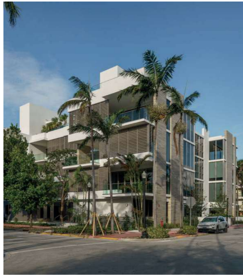
Louver House, Miami, USA
